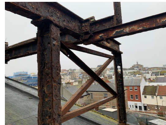
Photographs showing condition of steelwork in structure proposed for removal.
