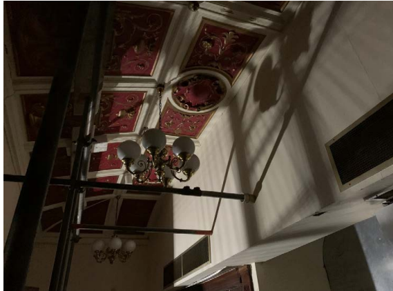
Mecca Bingo installed stud and plasterboard panelling masking heaters, ceiling and door surrounds
