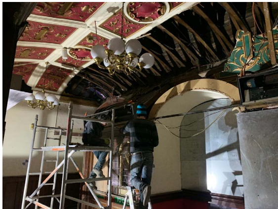
Vaulted ceiling and door surrounds exposed after removal of studwork
